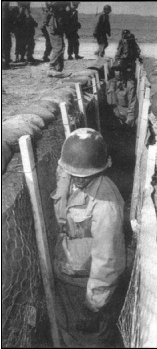
31. Observers entering trenches at the test site.
